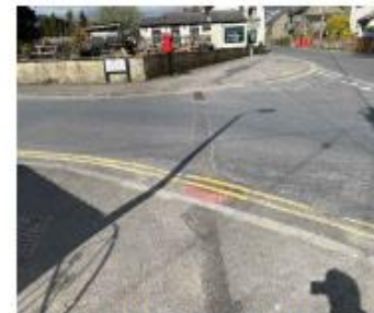
Existing dropped kerb / informal crossing point. May require tactile paving to be provided.
